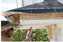
Roof overhangs, also known as eaves, can be finished in a number of materials—including PVC, wood, or aluminum. They can add a unique touch to a home exterior and are often a critical part of effective roof venting.
